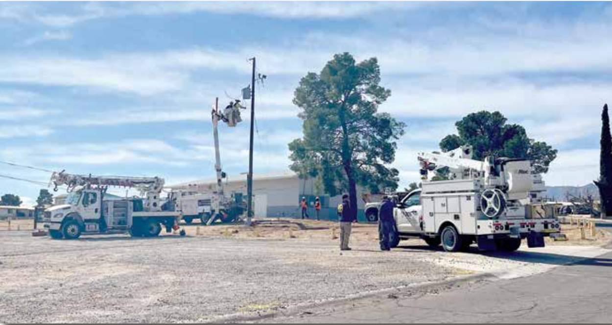
APS crews and contractors working on power lines and replacing light poles at the San Manuel Community Center and City Park. T.C. Brown | CANP
